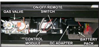
Figure 16.2 Valve Components
